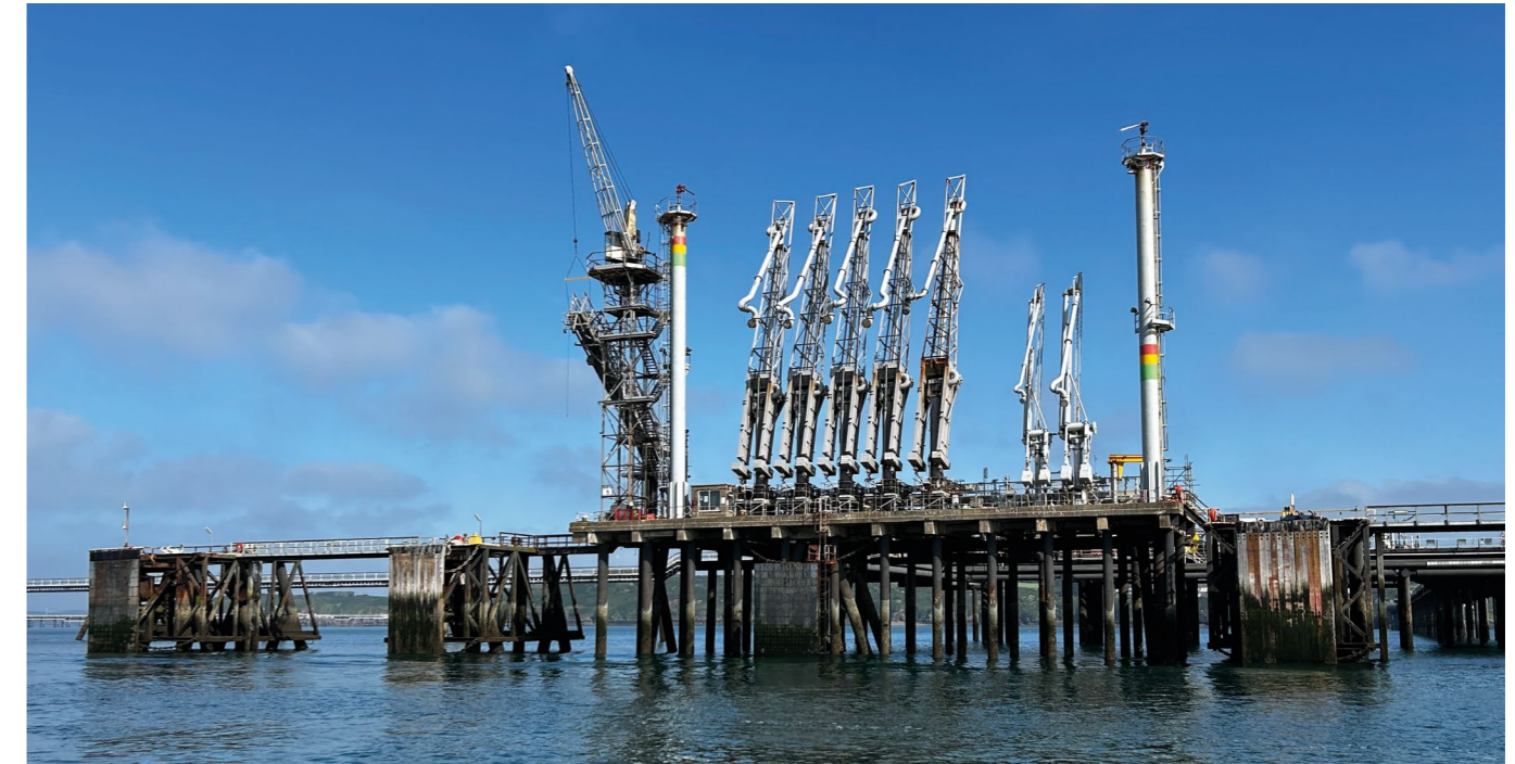
Figure 11 Liquefied gas loading/unloading arms at Milford Haven
