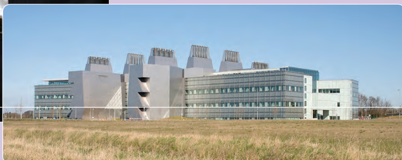
Photo: The new MRC LMB building, completed in 2013. Source: LMB
